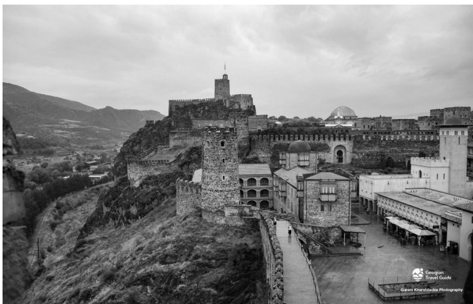
c12. Contemporary reconstruction of Akhaltsikhe fortress – the Rabat. 12
